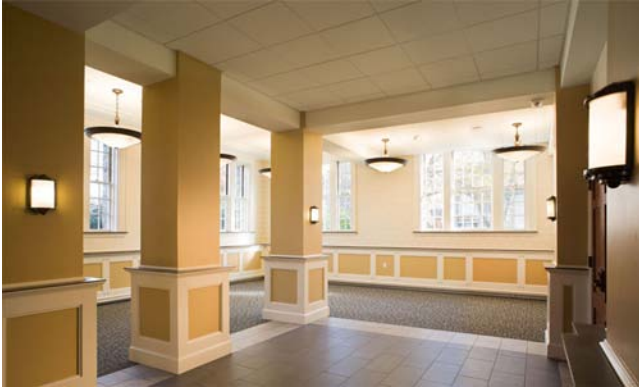
FIGURE 14. Theatre Sconces, MDF millwork, Corian sills.
