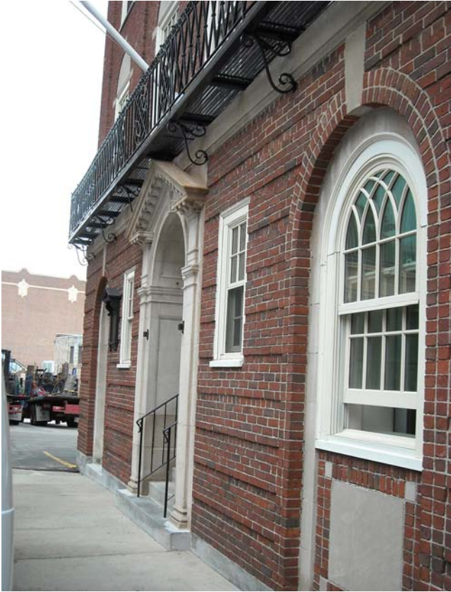
FIGURE 1. Historic façade salvaged.
